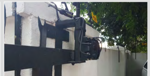
a+b. In-Line assembled Gate Contact
